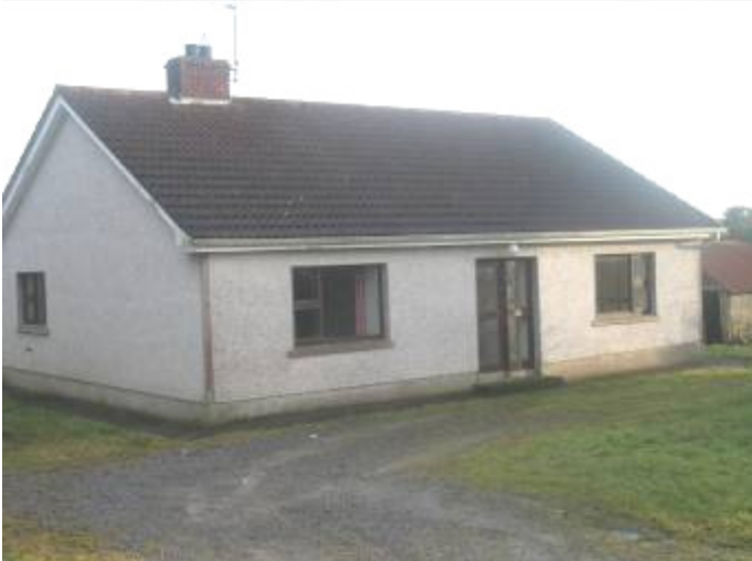
Front of Property
